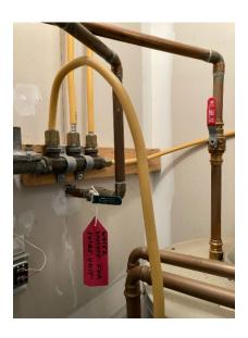
Below is a picture of what the shut off valve looks like in a Birches unit (50 houses). If you need to shut off the water – turn both valves vertical to shut off the water in your unit.
